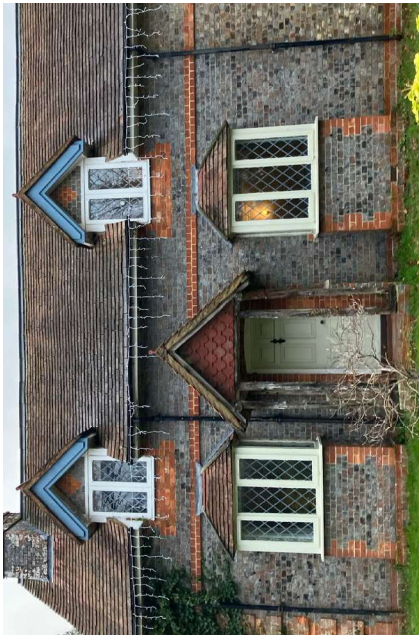
Figure 103: Example of highly ornamental brick facade with hung tiles and slate roof tiles, timber porch, brick quoins and windows with diamond mullions, Ifold.
