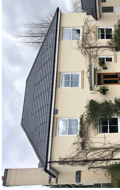
Figure 168: Use of shingle-like solar panels on a slate roof, with the design and colour of the solar panels matching those of the adjacent slate tiles.
