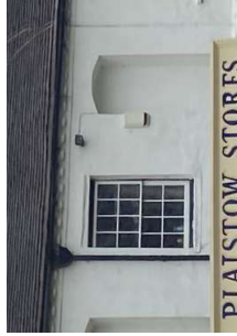
Figure 24: White sash windows with mullions.
